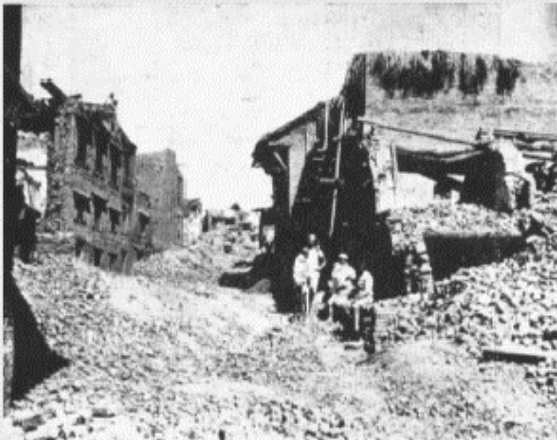
Damage caused by earthquake
