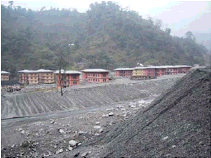
Housing colony damaged due to flash flood in Phuentsholing - 2000
