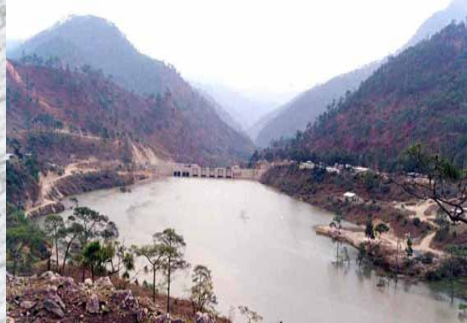
Kurichhu Hydropower Plant
