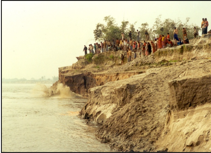
River Bank Erosion
