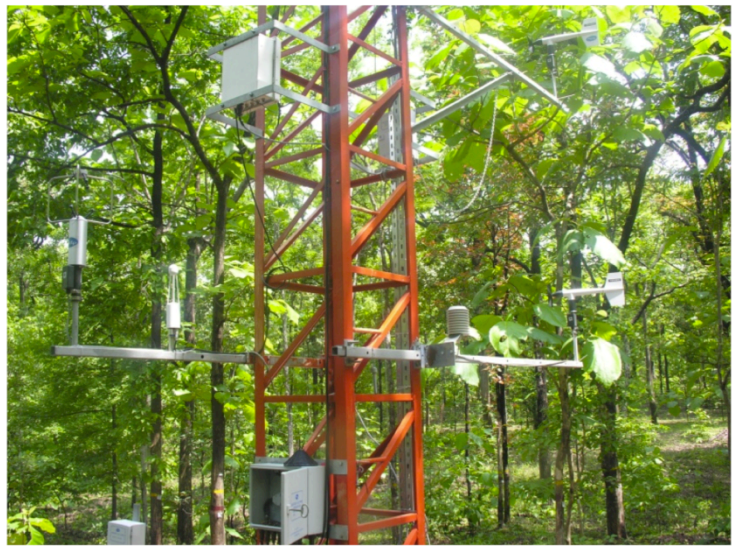
Betul Tower, Sonic anemometer, IRGA CO 2 /H 2 O analyser, (Fast sensors); Hygrometer and anemometer, (Slow sensors) at the lowest height
